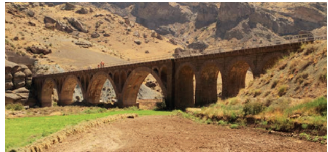
Fig. 2 A view of 475 Bridge
