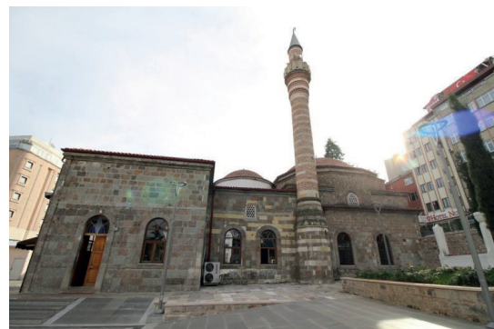
Fig. 11 Historical minaret of Iskender Pasha Mosque [48]
