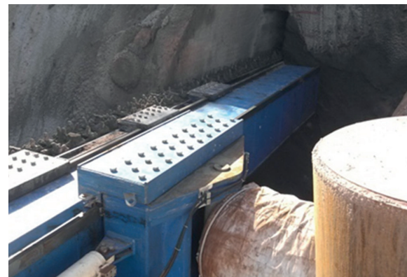
(b) The application of pre-cutting machine
