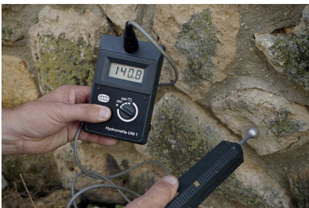
Fig. 12 Estimation of the structural moisture content with Gann-Hydromette Uni device
