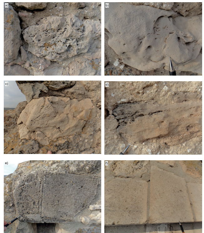
Fig. 5 Limestone masonry elements: (a) cemented macro-porous limestone; (b) sandy limestone; (c) highly cemented and cross layered limestone; (d) sandstone; (e) porous oolitic limestones (former replacement stone); (f) porous limestone (new replacement stone)
