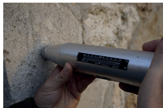
Fig. 10 Surface testing with Schmidt hammer
