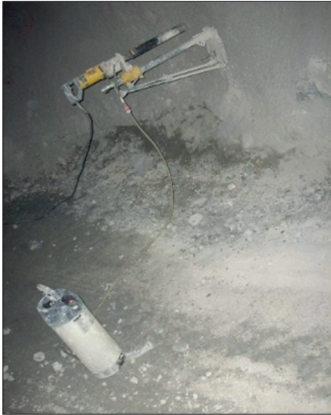
Fig. 2 The core sampling from shotcrete practiced in underground
