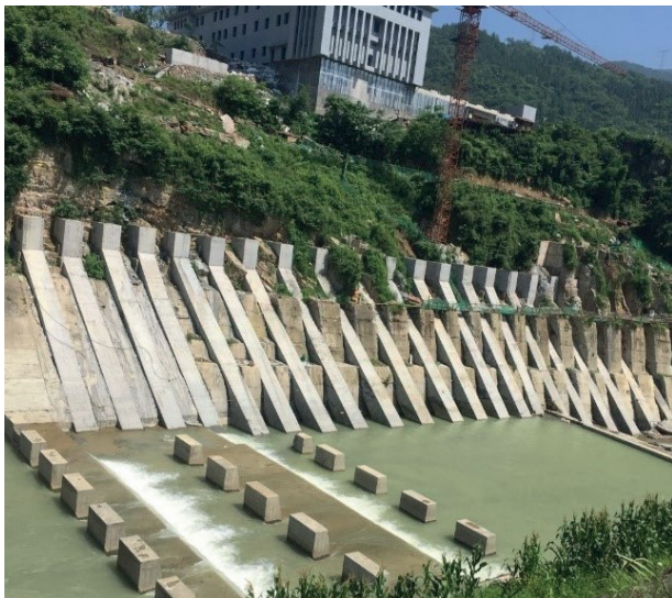
Fig. 1 Photograph of the slope (after reinforcement)
