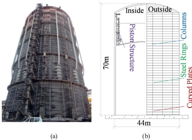
**Fig. 1** Investigated storage furnace gas (AFO) tank [13];
