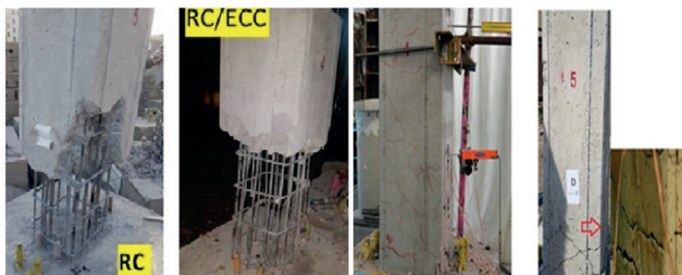
Fig. 11 Failure patterns of SP4 and SP5
