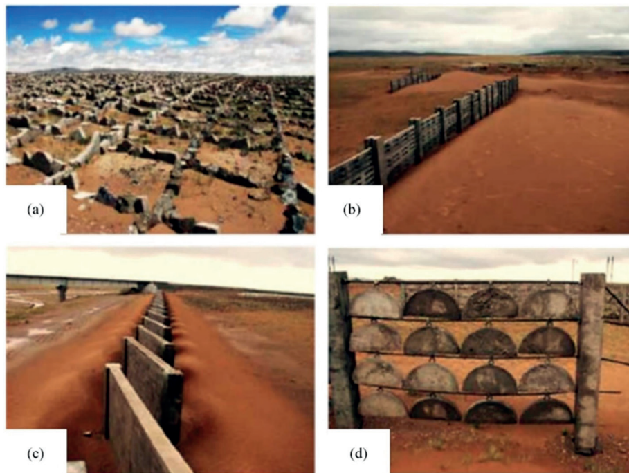
Fig. 2 a) Rocky checkerboard sand barrier; b) sand-blocking fence; c) sand-deviating board; d) wind-weaken leaf [8]
