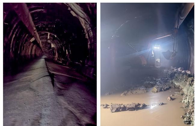
Fig. 2 The photo of the interior of No. 3 branch tunnel; (a) Upper arch deformation, (b) Subgrade excavation
