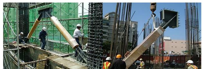
Fig. 2 BRB installation in RC frames
