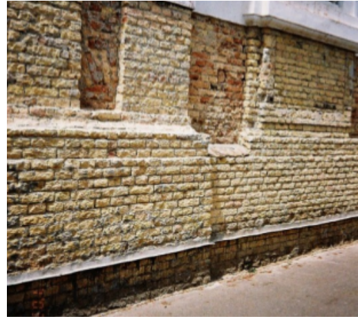
Fig. 20. Finished rising damp handling
