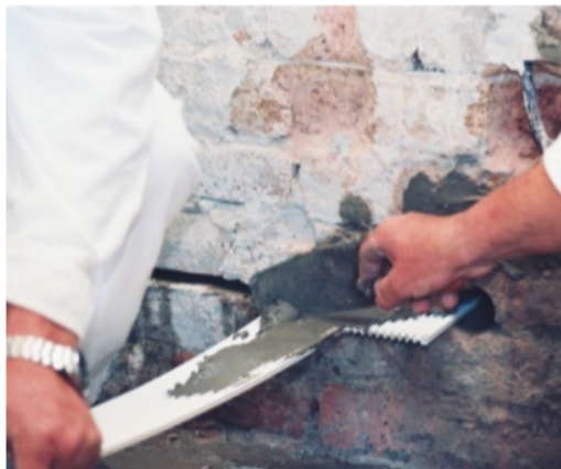
Fig. 19. Injecting the adhesion mass and Rail positioning
