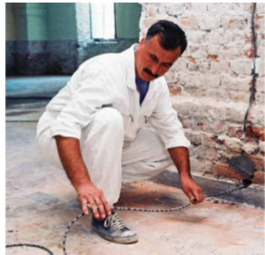
Fig. 15. Laying the cutter-cable
