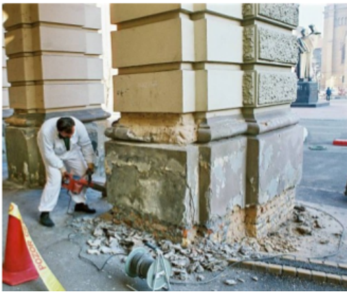
Fig. 13. Removing the mortar
