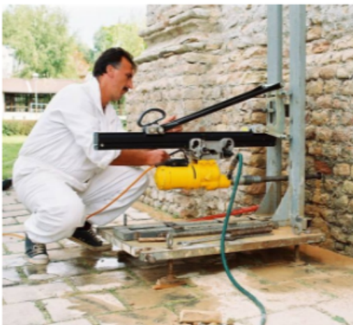
Fig. 14. Drilling holes
