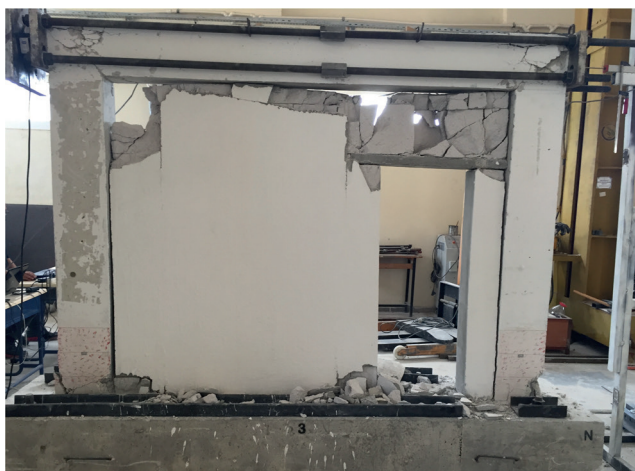
Fig. 27 (a) Crack map, (b) Failure pattern of RCF-4
