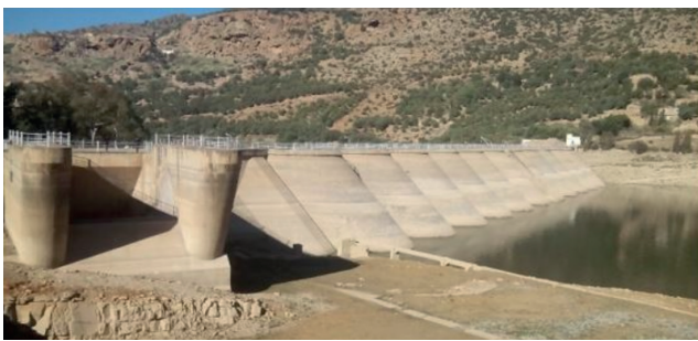
Fig. 1 Beni-Bahdel multi-arch dam
