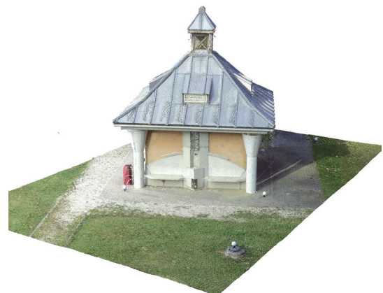
Fig. 1 Point cloud data of the small building
