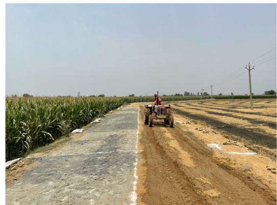
Fig. 5 Spreading of cement on the field sections
