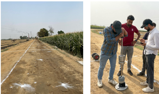
Fig. 8 Marking of points and conducting the LWD testing
