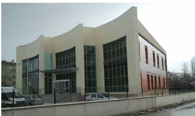
Fig. 3 The hospital building
