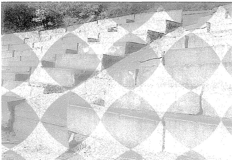
*Fig. 22.* Landslide and following creep displaced and fractured concrete seats at 'Vasas' sports ground
