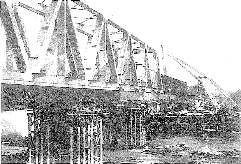
Fig. 8. The entire trussed bridge structure during assemblage
