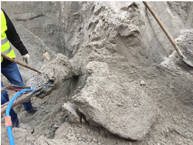
Fig. 3 Irregularly shaped masses found near the grouted anchors body
