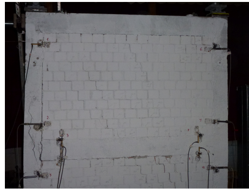
(b) Typical cracks on specimen
