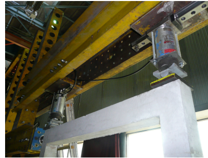
(b) Hydraulic jacks on an unfilled frame
