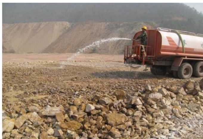
Fig. 1. Sprinkling water before roller compaction
