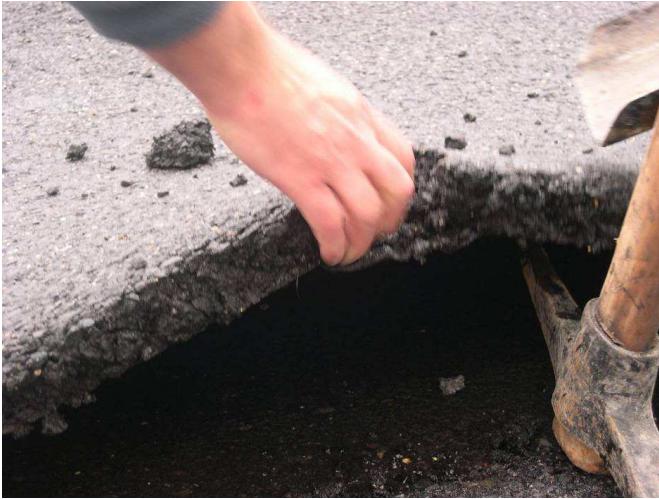
Fig. 1. An extreme example: because of the net usage there is no cohesion between the layers
