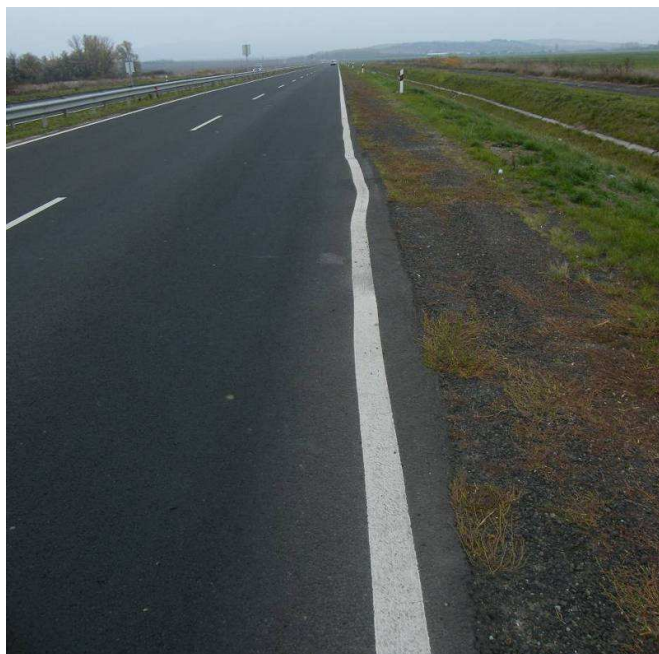
Fig. 2. Because of the build in tissue net, the abrasal layer slipped and a rut has appeared (route 21.)
