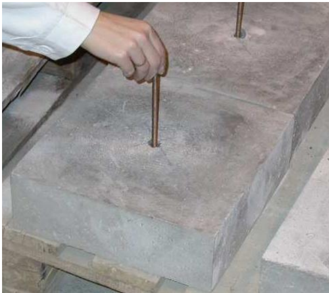
Fig. 6. Installation of the anchors
