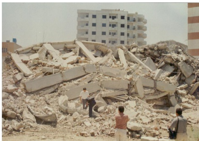
Fig. 1. A completely collapsed building in Kocaeli Earthquake [3, 4]
