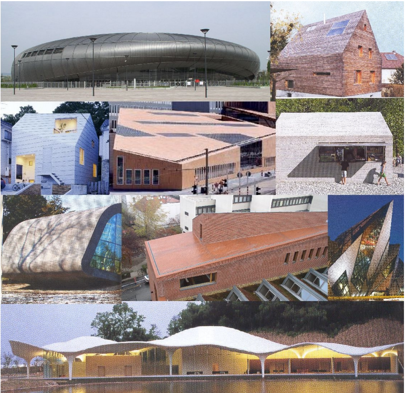
Fig. 1. Examples of buildings with covered roofs: variations of materials and shapes
