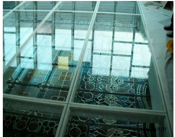
Fig. 15. Loadbearing "Kossuth, and Andrassy-bridge" Glass Slabs in Gresham Palace, calculations by K. Pankhardt, in 2002
