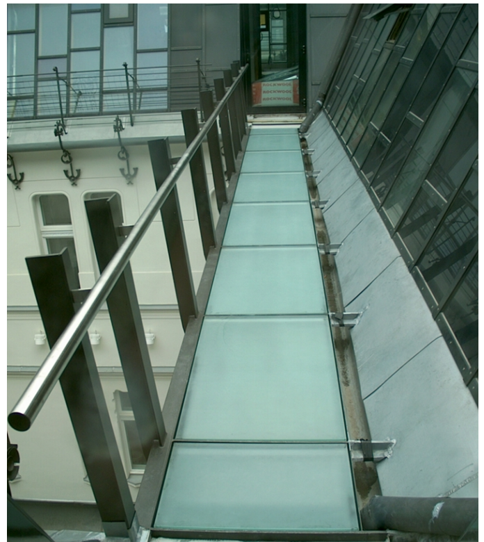
Fig. 16. "Gresham-bridge" cable tensioned bridge in Gresham Palace, calculations of glass and steel construction by K. Pankhardt, in 2002
