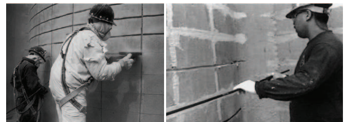
Fig. 12. Groove cutting and doweled of the FRP into a common wall [19]
