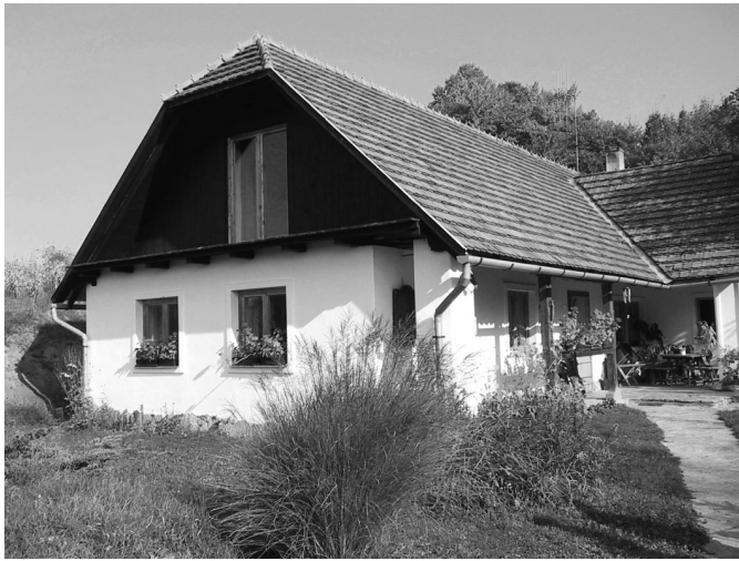
Fig. 3. The appropriate using of local materials: the background dwelling was built using the mud excavated from the nearby road. (Beaten –earth structure). This excavation opened the site, and created a new pathway for the tenants. Rural dwelling in Abaliget shows the good example of contemporary architecture and the tradition of local building history.
