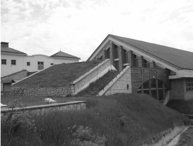
Fig. 2. Secondary school for Environmental studies in Tokaj: green grass roof solving as ecological pathway to study the native plants
