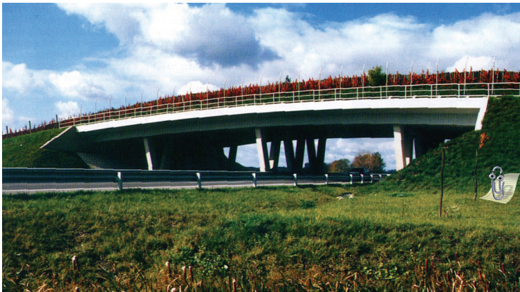
Fig. 2. Game bridge over motorway M1
