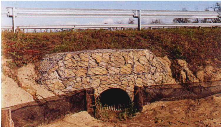
Fig. 4. One of twelve amphibian tunnels built under motorway M3
