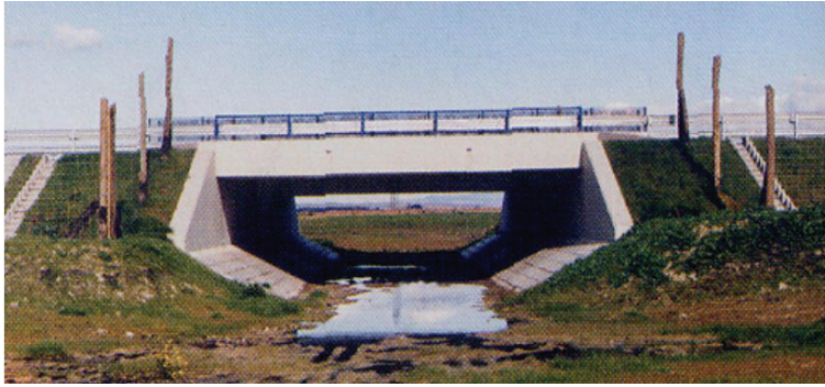
Fig. 3. Game passage-with guiding fence-under motorway M3
