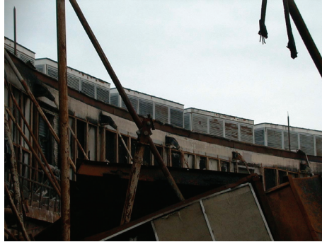
Fig. 7. Destroyed cable heads [4]
