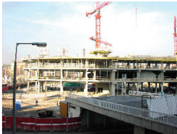
Fig. 4. The Budapest Sports Hall under construction (1981) ( www.index.hu )
