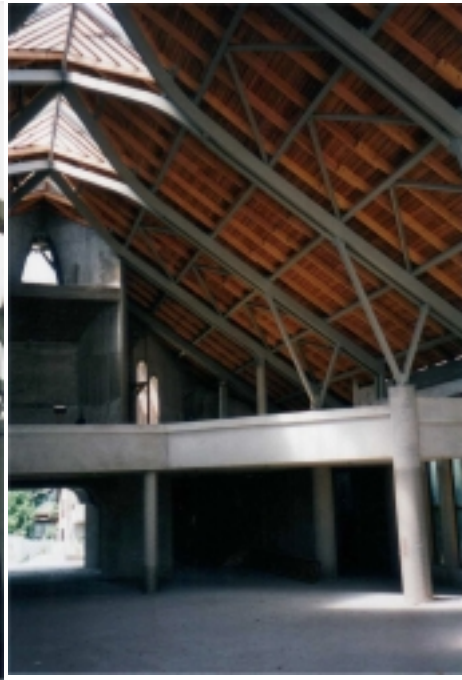
Fig. 8. The structure of the roof
