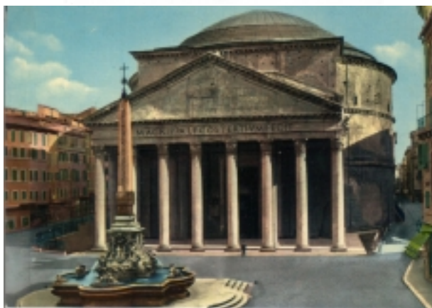
Fig. 2. The Pantheon in Rome: A) Structural section and plan (Renaissance drawing) B) Main façade
