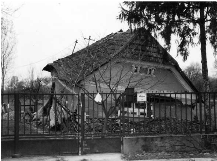
Picture 2. Example for collapsed loam house because of the floods of River Tisza
