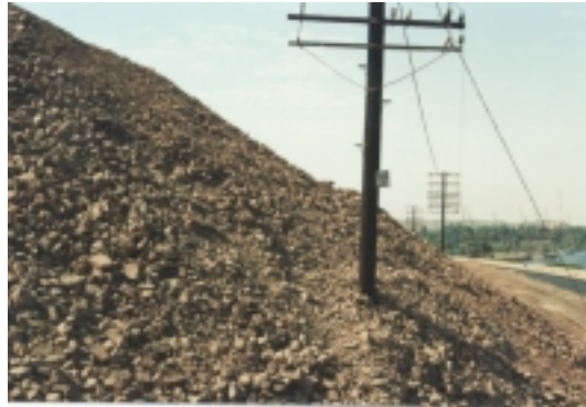
Fig. 19. Sandstone debris form steep slopes alongside the railway track, section 855+500
