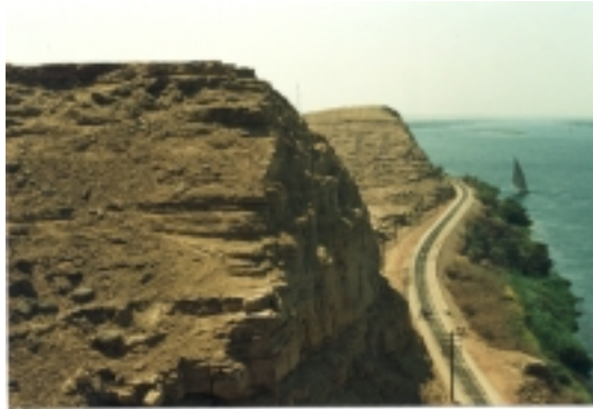
Fig. 8. The railway track is bordered by steep cliffs to the W and by narrow vegetated land on the riverside of Nile to the E
