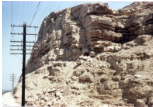
Fig. 10. Detail of the densely jointed cliff face. The joints are parallel to the railway track, 793+520 section
