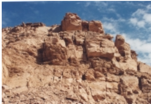
Fig. 18. Railway track perpendicular joints in the cliff of the section 854+300
