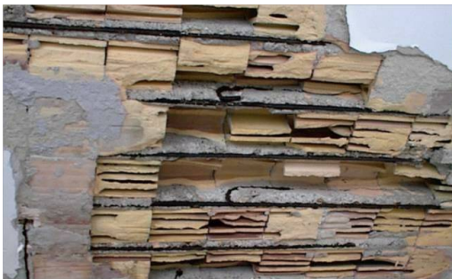
Fig. 3. Appearance of the ceiling
