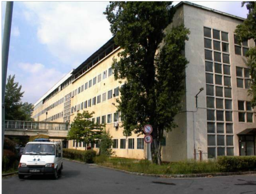
Fig. 2. The building in which the discussed failure occurred
