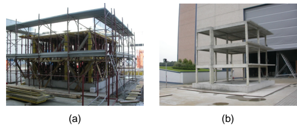
Fig. 14. Scaled specimen (a) during and (b) after construction
