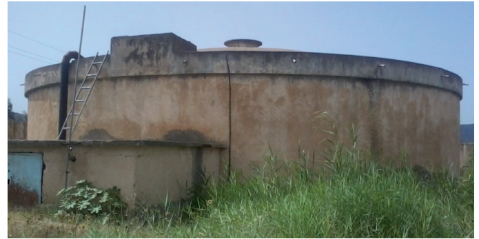
Fig. 2 General view of Touares tank
