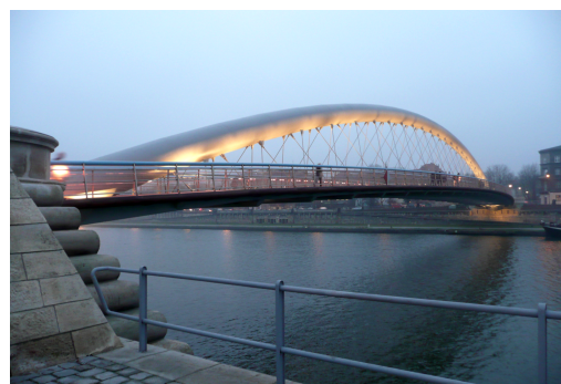
Fig. 5. Side view on the Father Bernatek footbridge in Cracow
