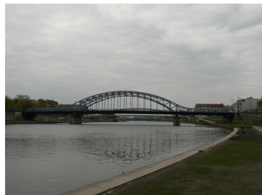
Fig. 3. Side view on the Marshal Jozef Pilsudski Bridge in Cracow
