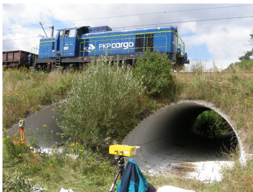
Fig. 4. Side view on CSP railway culvert in Krosnowice during tests
