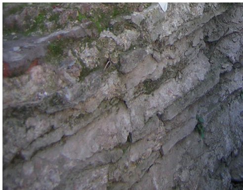
Fig. 2 The brick-mortar walls of the building
