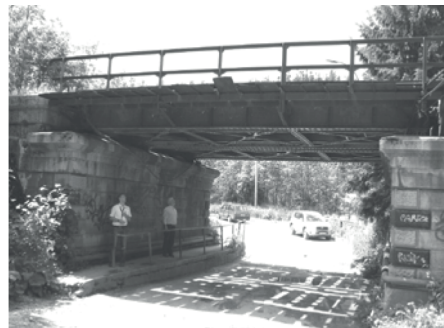
Fig. 20 Railway underpass; span L = 8,60 m.
