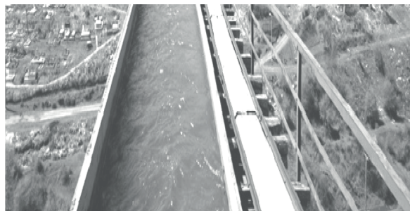
Fig. 12 Aqueduct Reșița, after refurbishment
