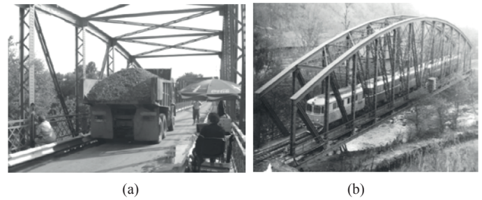
Fig. 5 In situ tests on bridges: (a)-highway bridge; (b)-railway bridge
