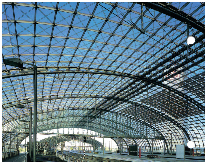
Fig. 1 The train station (Lehrter Station in Berlin), an example of the glass-aluminium shell structure
