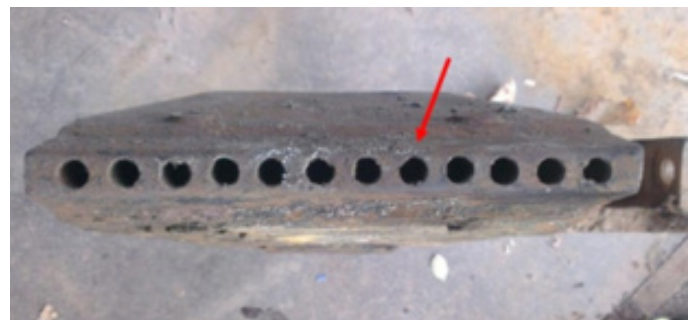
Fig. 11 MONTAZER GHAEM boiler fuel torches
