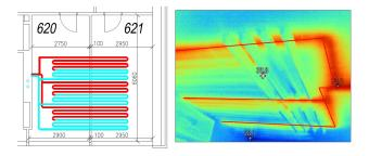
Fig. 4 Heating pipes in ceiling determined by thermocam (1 – hydraulic separator, 2 – circulator pump, 3 – three-way mixing valve)
