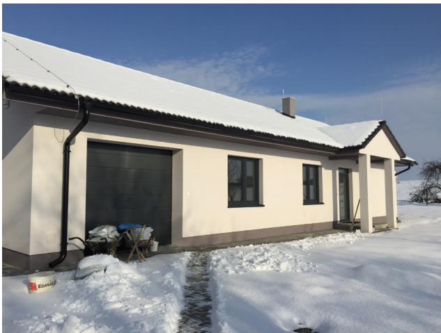
Fig. 1 A real view of the house
