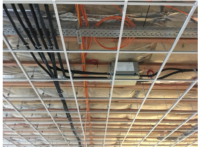
Fig. 9 Indoor unit installation (authors' archive)
