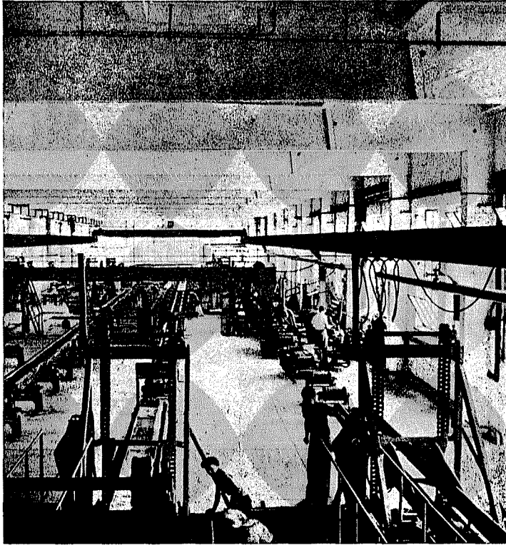
Fig. 6. Photograph of prestressed concrete sleeper manufacturing plant at Lábatlan
