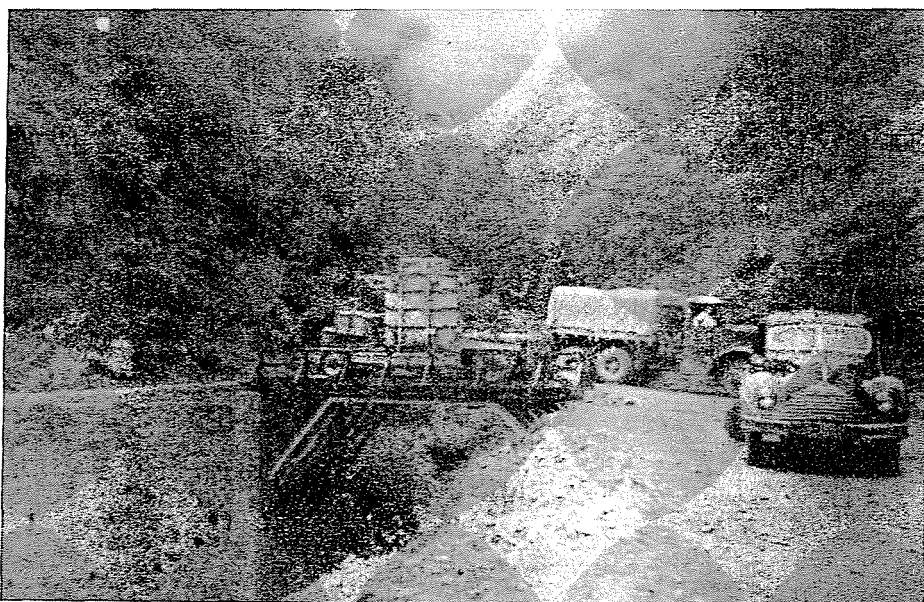
Fig. 13. Transport of transformers through the mountains
