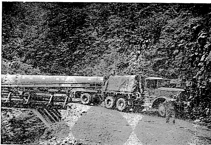
Fig. 12. Sharp curves caused problems for long pipes
