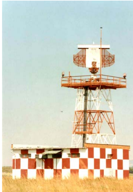
Fig. 6. SELANIA ATCR-33 radar building and its aerial
