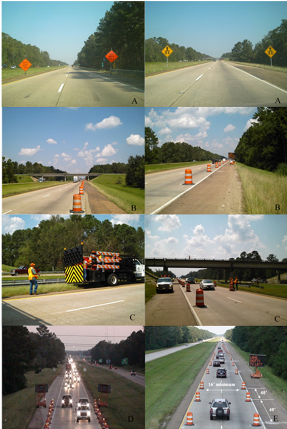
Fig. 4 Set up Progression of a Two-Sided Taper (a) static signs (b) closed lane tapers (c) open lane-opposite side tapers (d) beacon lights (e) channel device spacing
